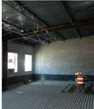
The multipurpose room was added on the north side.
